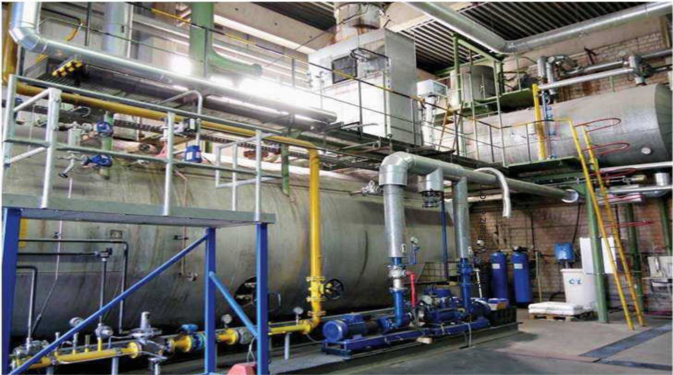
② Steam boiler in the boiler room at Kunert Wellpappe in Biebesheim.
