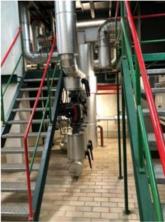
An example here involves the use of a heat exchanger for the conversion of surplus steam into hot water at a temperature of 80°C (figure 2), which is used for heating purposes and the return of any further surplus in the form of condensate to the steam power plant.
