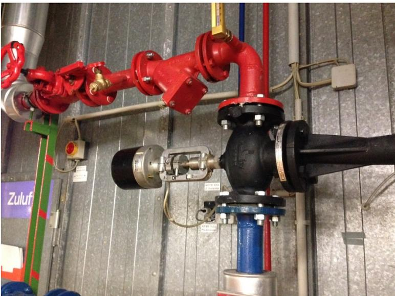
**Figure 2** Ejector installed in a building at the Free University of Berlin in 1977
