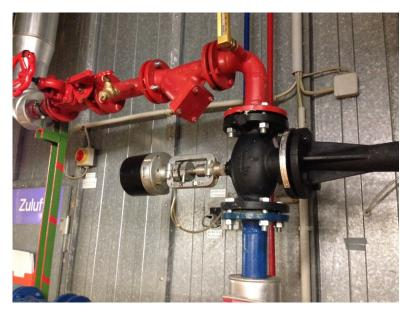
Figure 2 Ejector installed in a building at the Free University of Berlin in 1977
