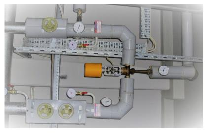
Figure 5 Ejector with air register in the example
