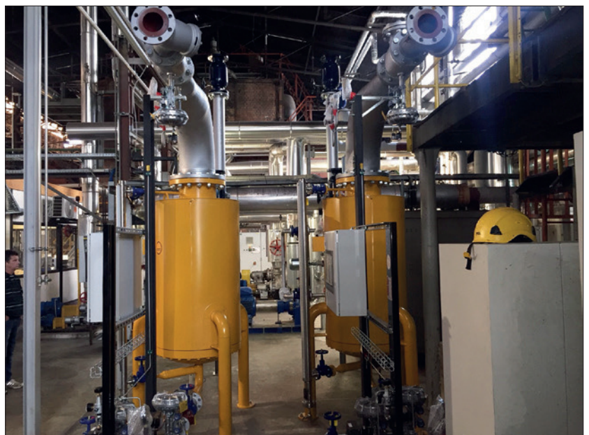
Figure 2. Two steam-water heat exchangers in sequence
